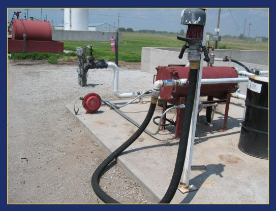
Check hoses for evidence of blistering, weather cracking, carcass saturation or separation, cuts, nicks, or abrasions that expose reinforcement material, and for slippage, misalignment, or leaks at couplings.
