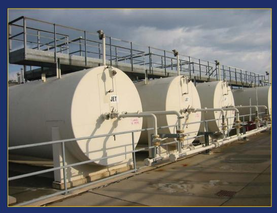
Above ground fuel tanks need to be grounded or bonded together and connected to a grounding rod.
