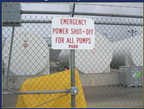
The emergency fuel shutoff system shall include shutoff stations located outside of probable spill areas and near the route that normally is used to leave the spill area or to reach the fire extinguishers provided for the protection of the area.
