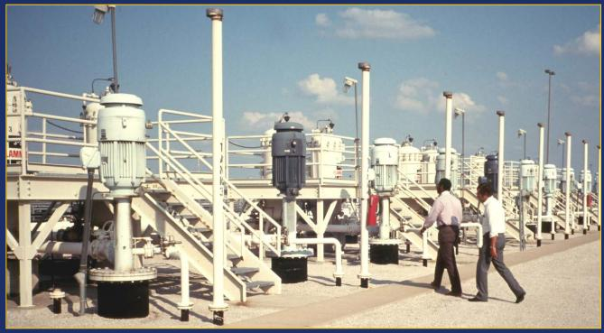
An Airport Fueling System is an arrangement of aviation fuel storage tanks, pumps, piping, and associated equipment, such as filters, water separators, hydrants and station, or aircraft fuel servicing vehicles, installed at an airport and designed to service aircraft at fixed positions.
